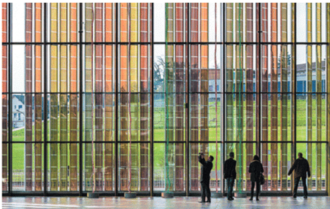
figure 2 . example of perovskite solar cells used in windows( http://news.sciencemag.org/node/112358 )
